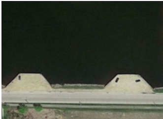
Upper Harbor Bulkheads
