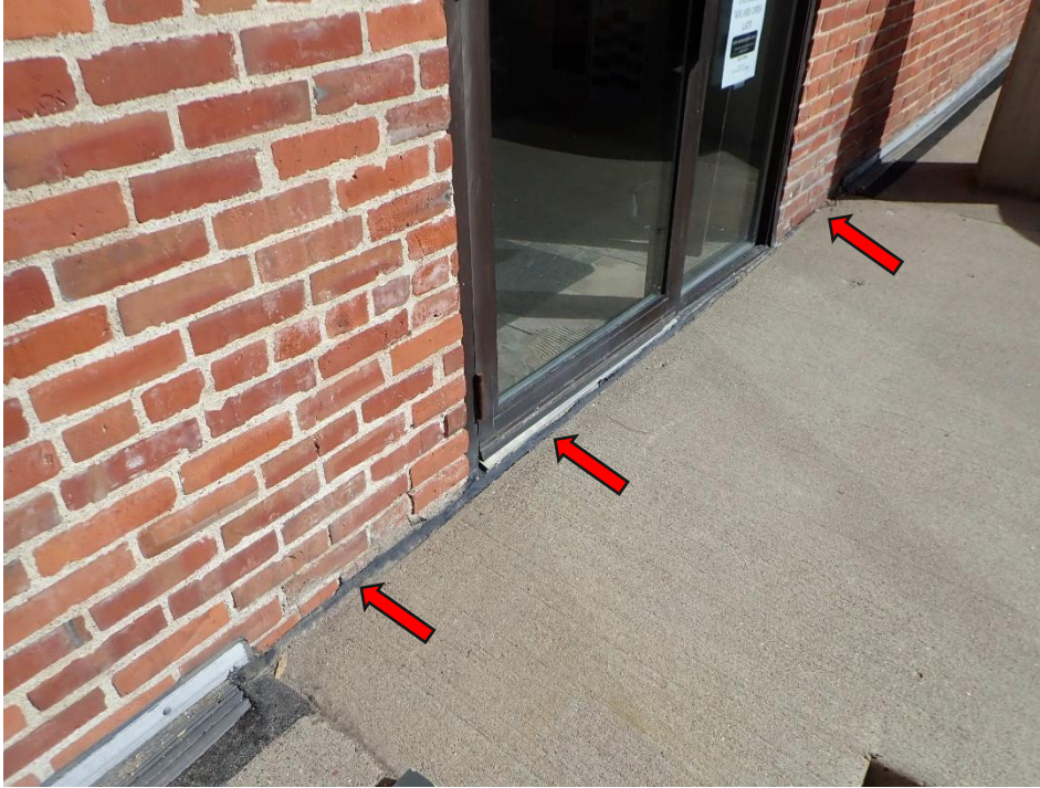
Photo 33. Typical isolation joint surrounding column base at the Lower Level which is open and leaking water to foundations/footings.
