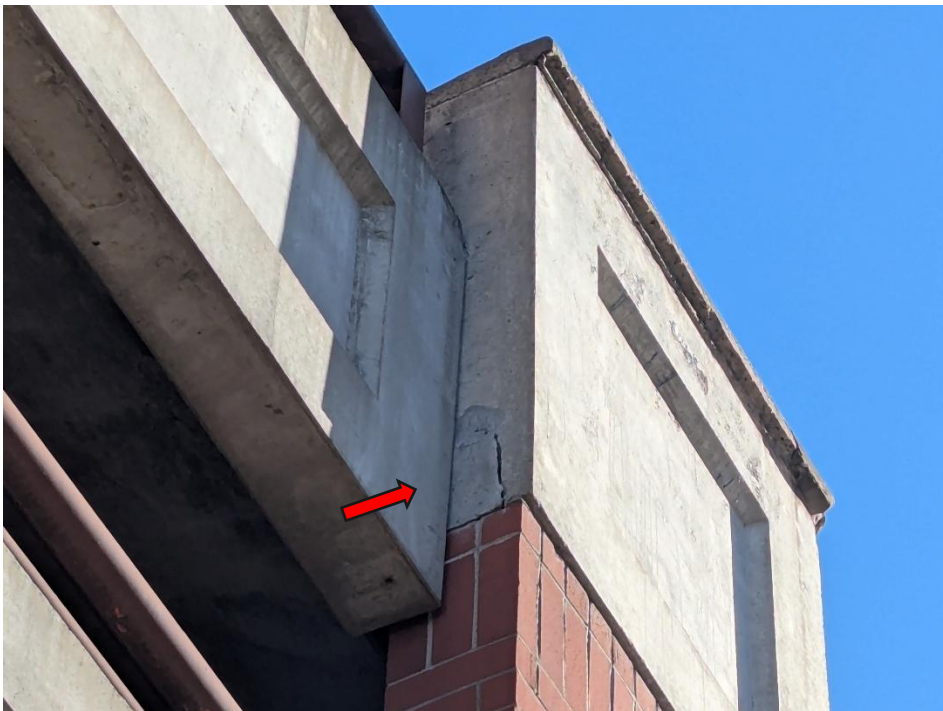
Photo 49. View of damaged and cracked precast concrete facade panel at the southwest corner of Level D from the exterior.
