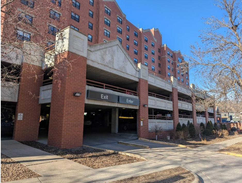
Photo 42. Overall view of the Seminary Parking Structure, south facade.
