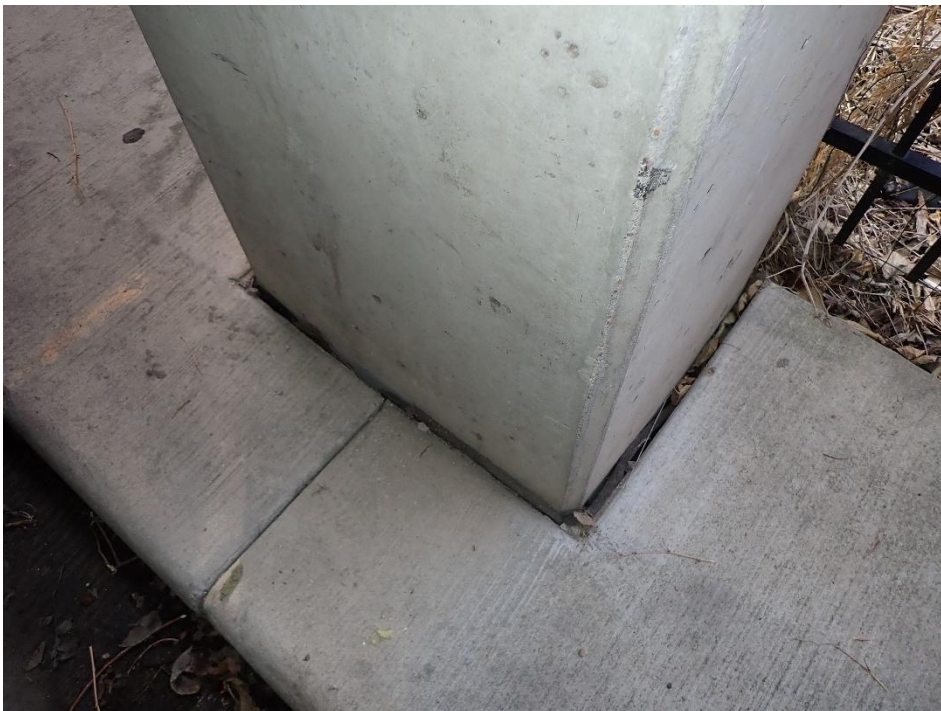
Photo 33. Typical isolation joint surrounding column base at the Lower Level which is open and leaking water to foundations/footings.
