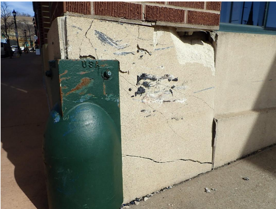
Photo 39. Close-up view of cracked and damaged precast facade panel at the northwest corner of the elevator tower.
