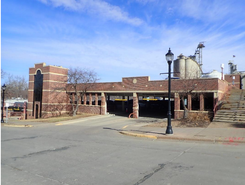
Photo 12. Overall view of the LaGrange Parking Structure, west facade.
