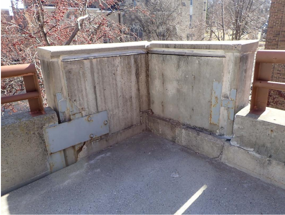
Photo 49. View of damaged and cracked precast concrete facade panel at the southwest corner of Level D from the exterior.
