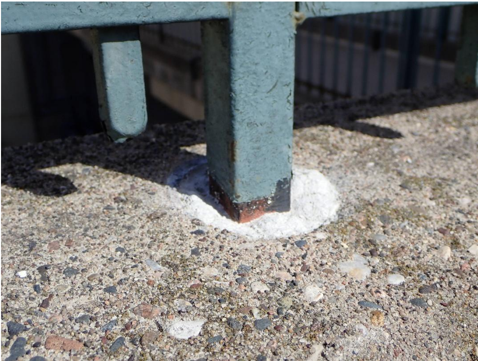
Photo 35. Close-up view of surface corrosion on steel pedestrian railing post at base.
