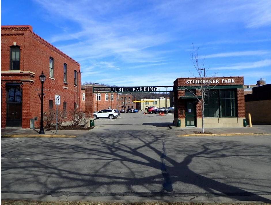
Photo 28. Overall view of the Studebaker Parking Structure, west facade.
