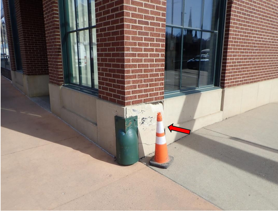
Photo 39. Close-up view of cracked and damaged precast facade panel at the northwest corner of the elevator tower.
