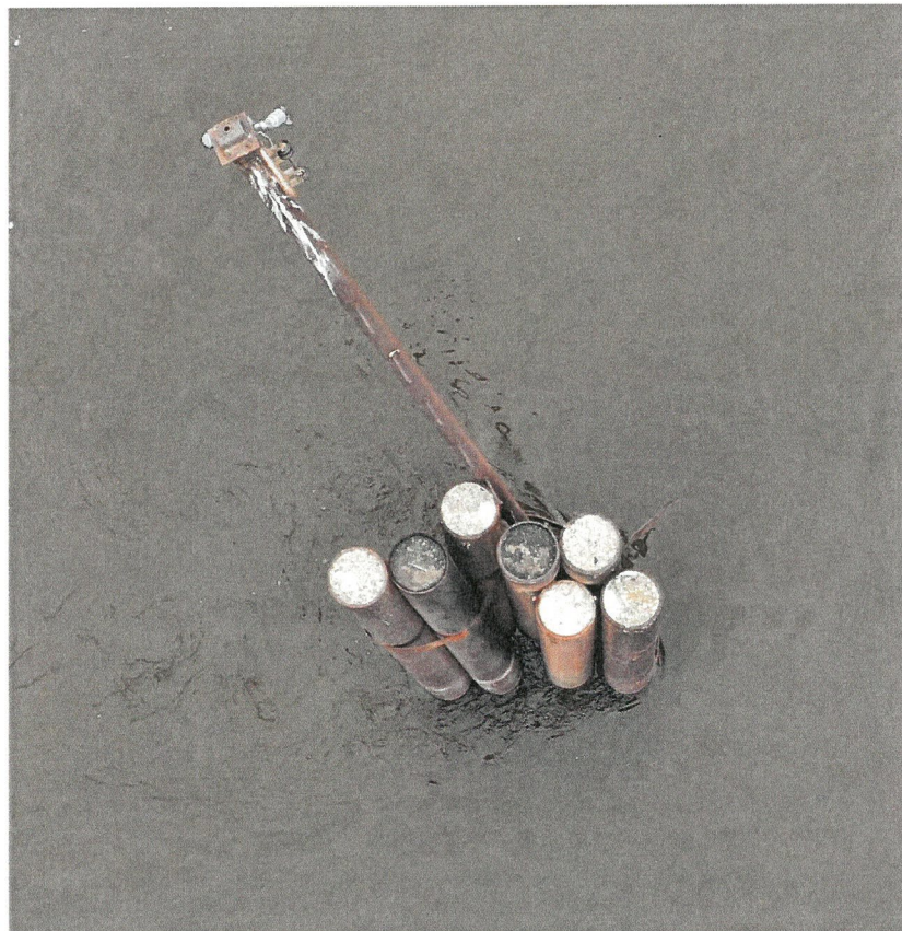
Figure 4. Dolphin #2 Aerial View
