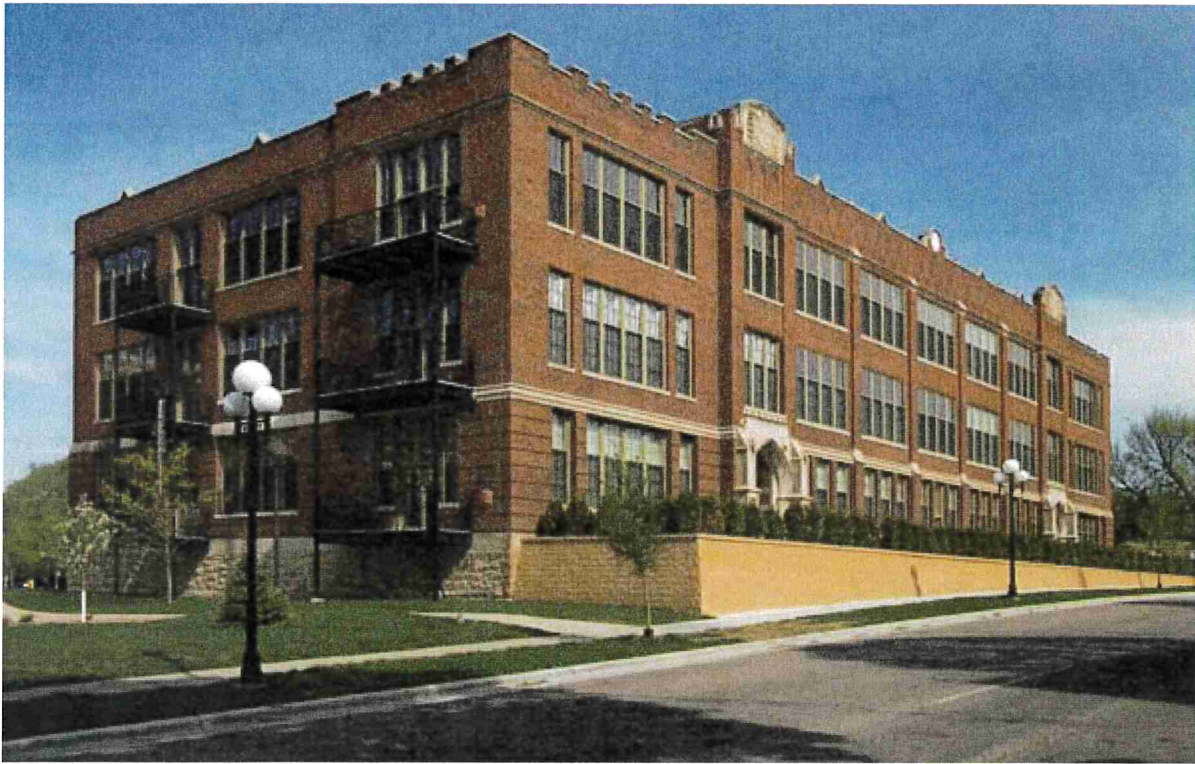
Central Park Condominiums (1916 Central High School) Downtown Red Wing, Minnesota
