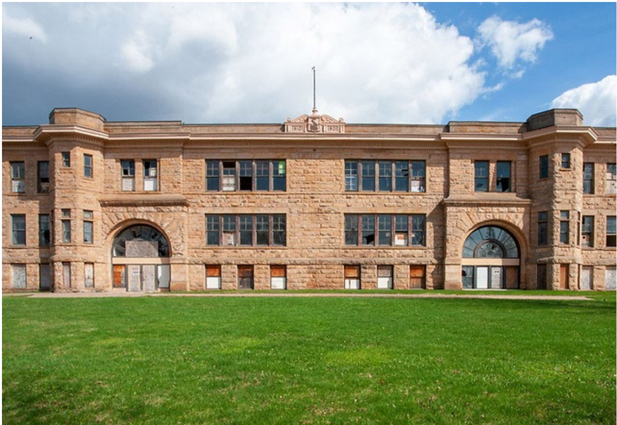
Construction underway for 'The Rock' housing project in Sandstone
