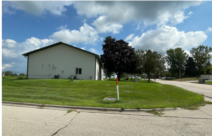
Examples of other buildings in the neighborhood
