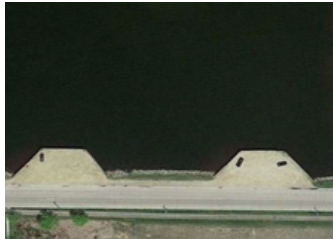
Upper Harbor Bulkheads
