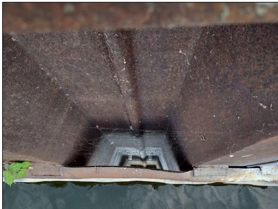
Figure 4: Existing Condition of Steel Rub Rails
