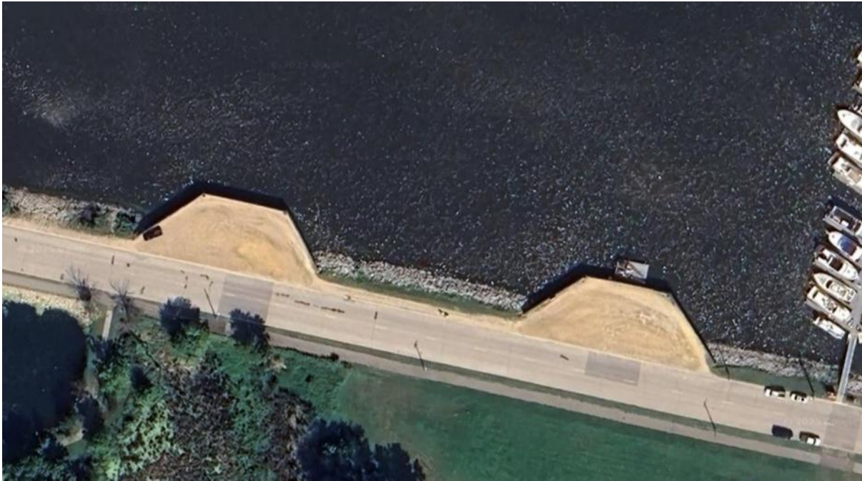
Figure 1.10: Upper Harbor Dock Wall (photo courtesy of Google Earth)
