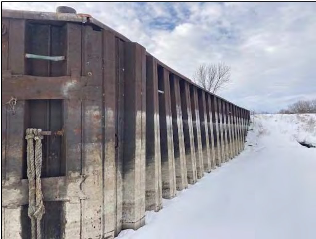
Figure 8: Condition of Dock Wall at STA 0+78 on West Bulkhead
