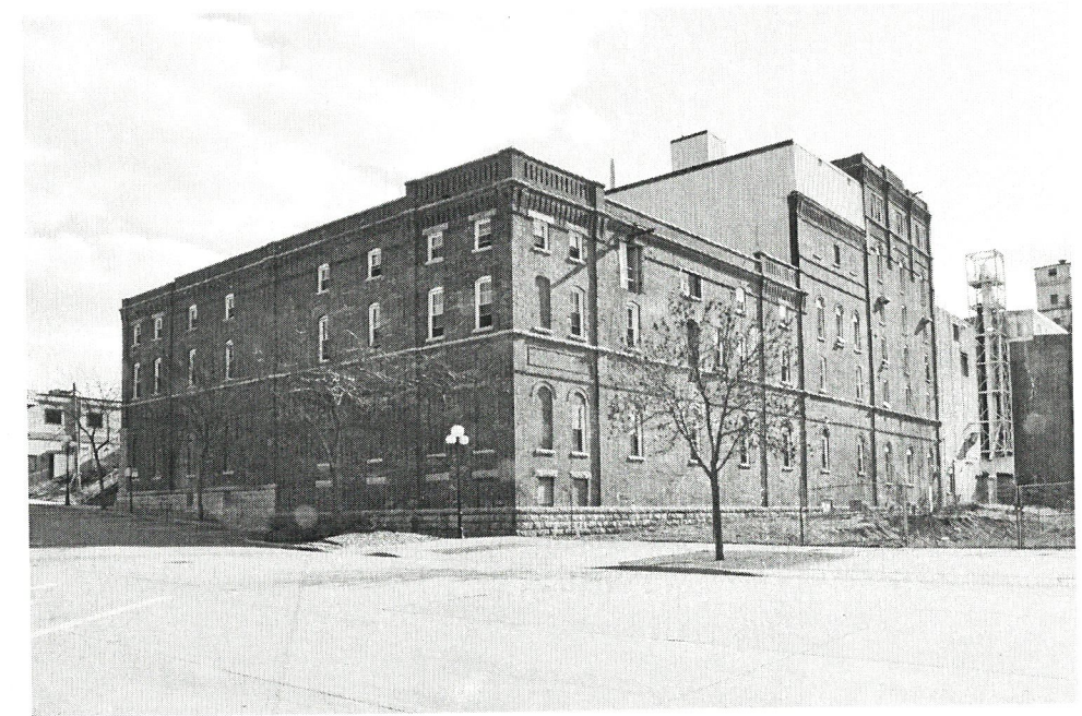
Fig. 211. 102 Broad St. Red Wing Malting Company, germinating and attemporating building, and the kiln house, which is the six-story brick structure (facing SW)
