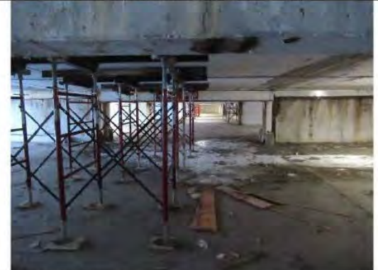
Photo 36: 7250 Parking ramp temporary shoring
