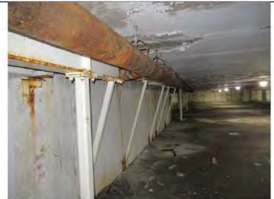
Photo 34: 7250 Parking ramp structural steel shoring
